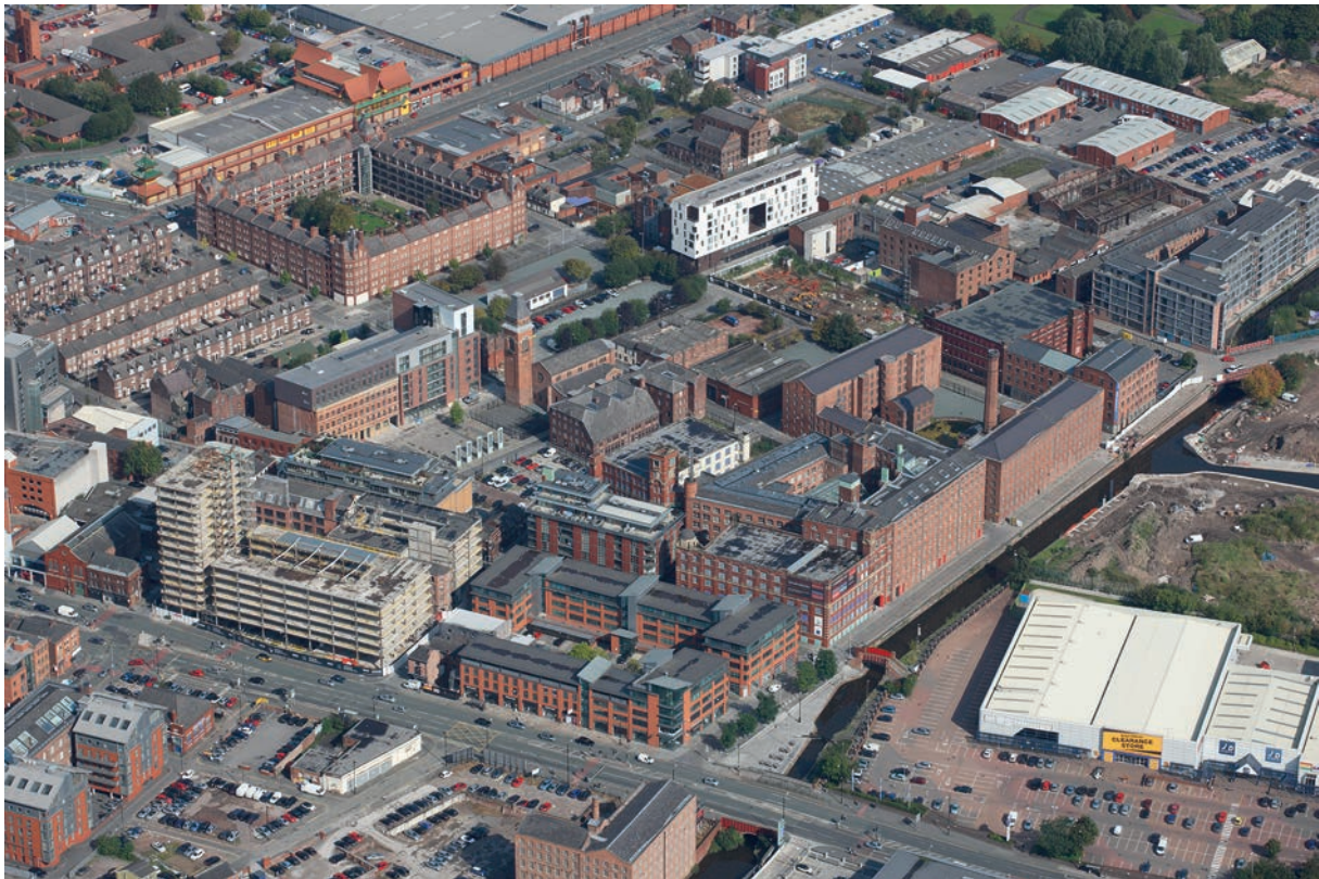
Figure 3b – aerial photograph of Ancoats taken in 2014
